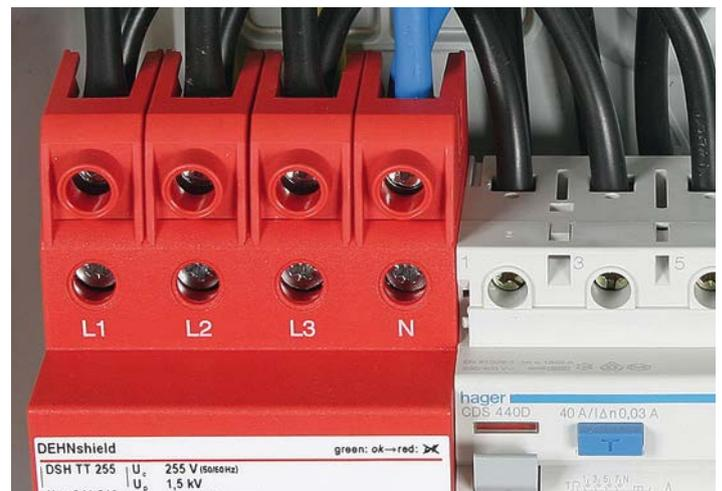
Figure 2: DEHNshield® with STAK 25 terminals
